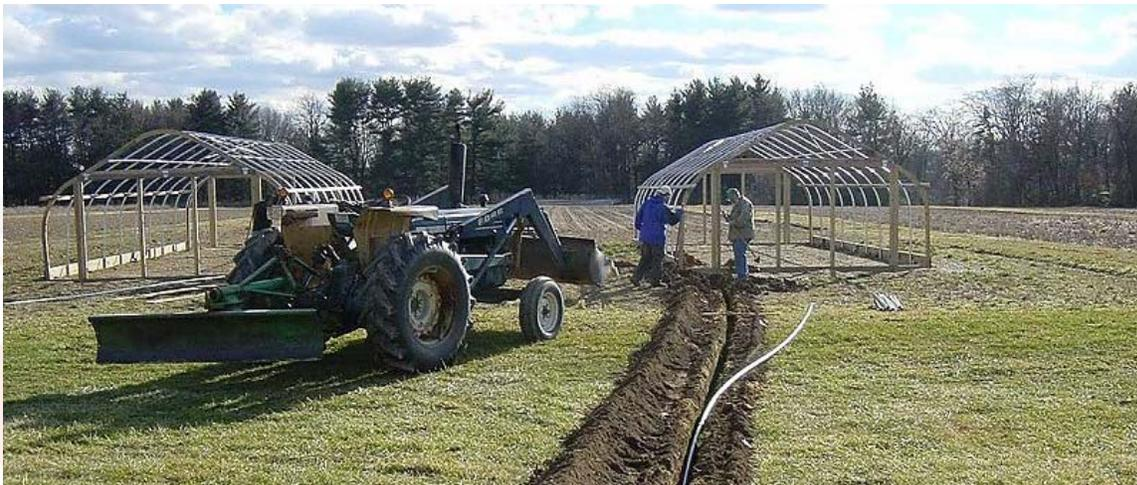
RCE agents demonstrate trenching of water and electricity to a high tunnel under construction
