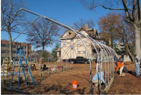
Construction of 20' x 36' high tunnel (EastPoint, Rimol Greenhouse Systems, Inc.) in East Orange. *Photo by A.J. Both*
