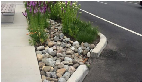
Rain gardens that create temporary ponds during storms will be constructed as part of the grant-supported project.
